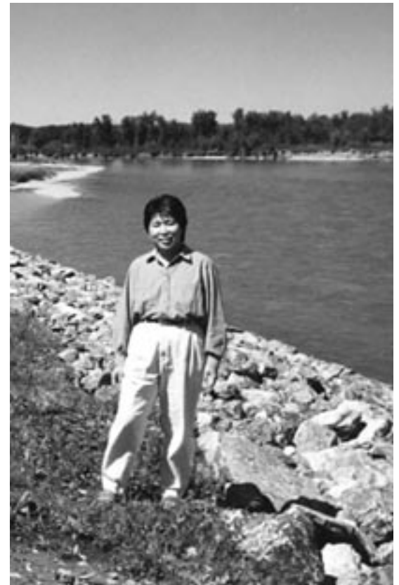
Bunny on site inspecting riprap protection along the Bow River bank, Siksika Nation (Blackfoot Indian Reserve).
